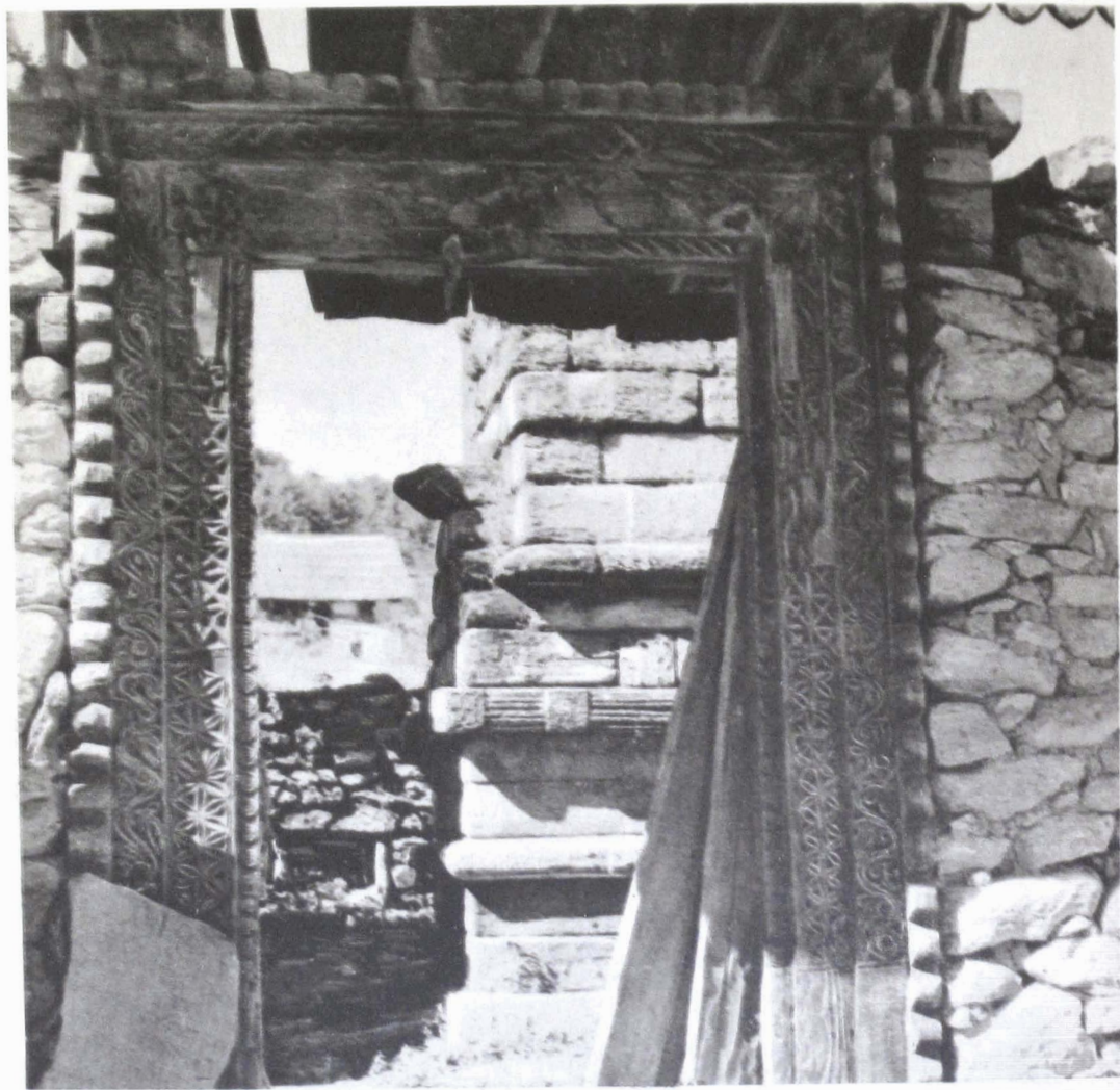
Fig. 39. Door of the enclosure surrounding the shrine of Chilkhā (p. 43)
